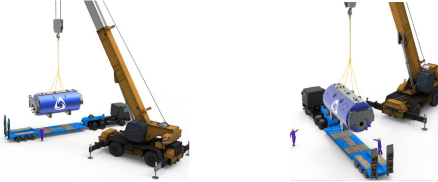
Figure 3.1.1 Placing Heater on Transport Vehicle
