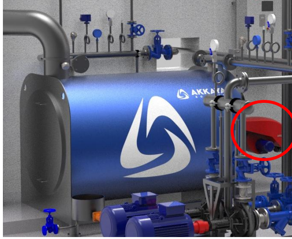
Figure Ap. 2.1 Burner on the Boiler
