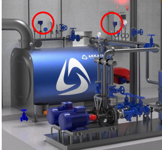
Figure Ap. 2.4 Pressure Switches
