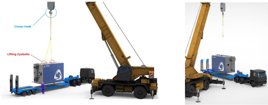
Figure 3.1.1 Placing Boiler on Transport Vehicle
