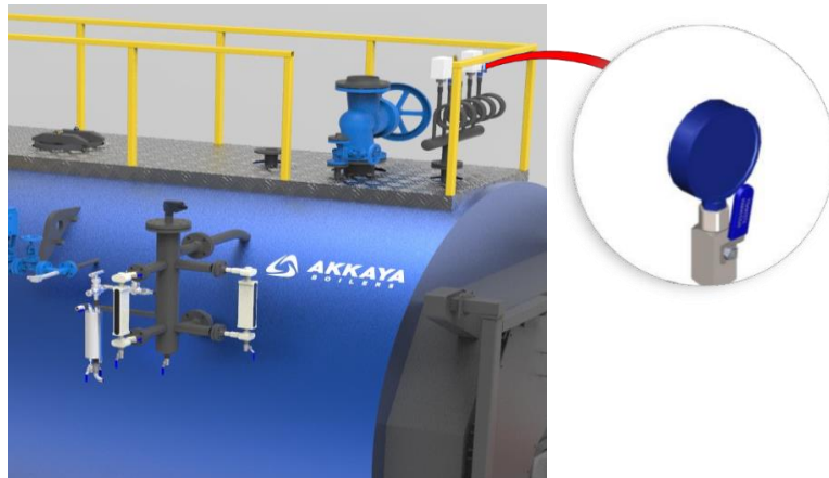
Figure Ap. 4.12 Manometer & Manometer Valves
