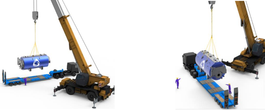
Figure 3.1.1 Placing Boiler on Transport Vehicle
